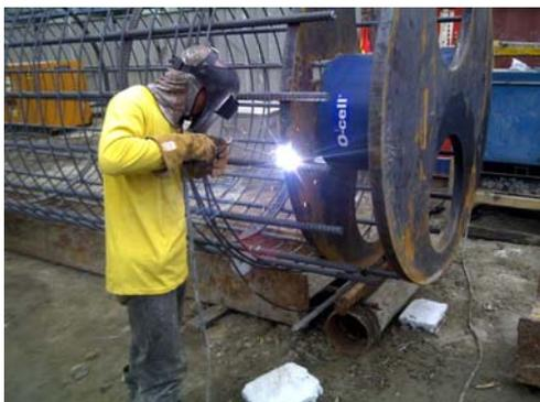
Attaching O-cell Assembly to Cage
